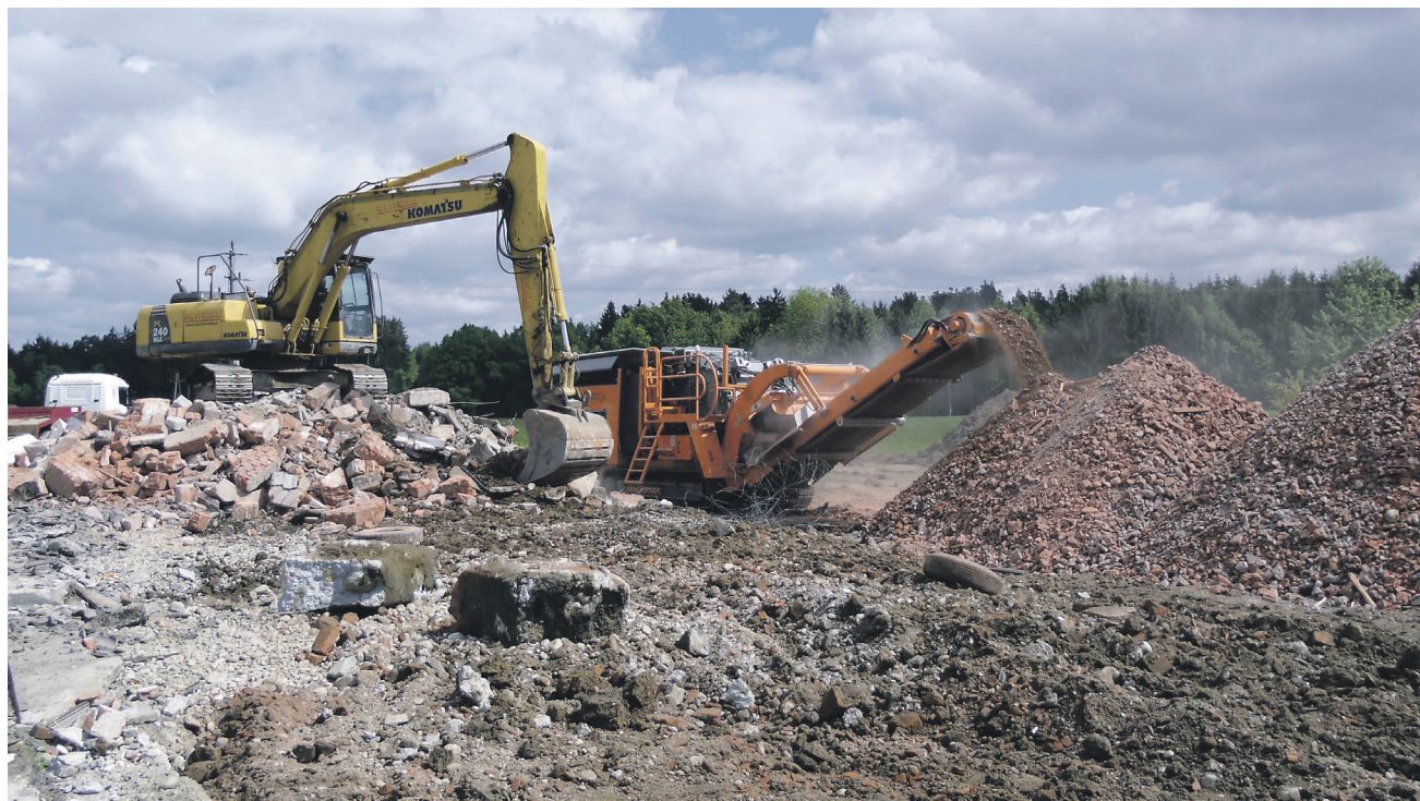
Rockster R900 Impact Crusher: Recycling of construction waste after demolition of a building.
