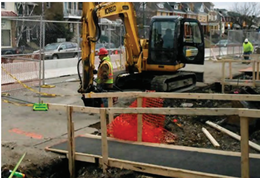
Where ongoing work allows for pedestrians to come and go from businesses that are open during working hours, the need for passage through the jobsite needs to be adequate. The sidewalk and ramp over the excavation are not up to ADA or MUTCD standards.
