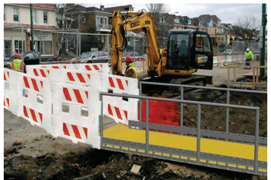
Proper barricading and ramp access is shown in place, providing safe access to and from the open businesses on this city street. PSS BoardWalk RAMP — a temporary pedestrian modular ramp — provides the necessary guidance for use of canes and walking devices.
