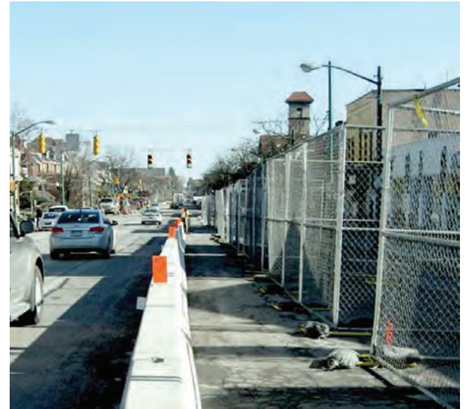
Right: There are trip and fall hazards (sandbags) at the base of the security fencing installed on the right hand (jobsite) side of the walkway.
