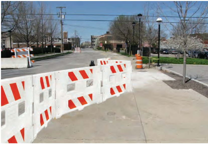
After: The left side of the hazard is protected with a continuous barrier.
