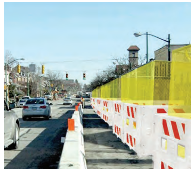
Continuous interlocking barriers are installed on the right-hand side of this temporary walkway to prevent trip and fall accidents.
