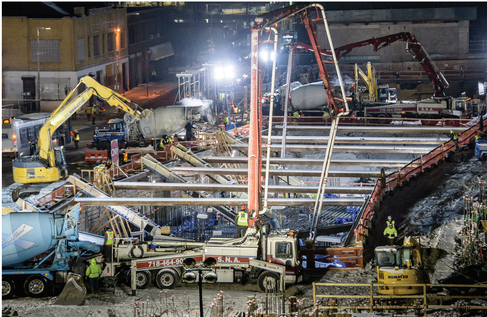
Six chutes were set up on 147th and 148th Streets with two pump trucks positioned on both the west and east sides of the site.
