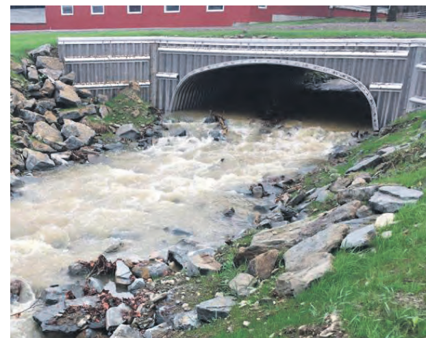
After: Culverts were replaced to the appropriate width, set at an elevation to promote natural streambed materials to fill the bottom of the culverts.
