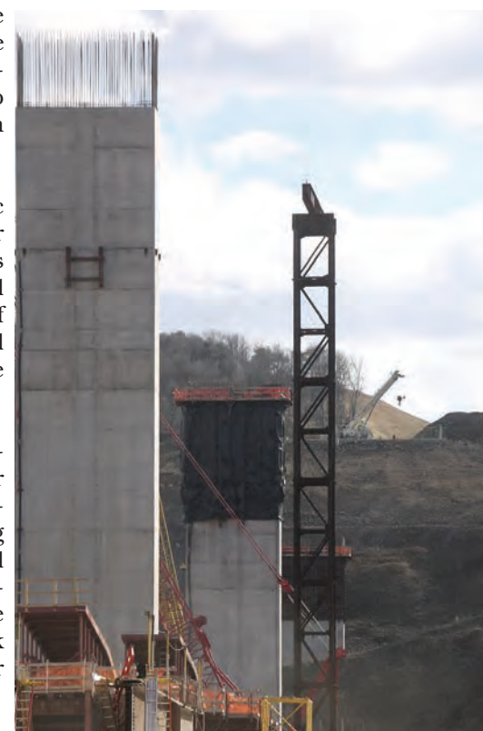
The second bridge pier is covered with plastic over insulation for proper curing of recently poured concrete at bitterly cold temperatures.
