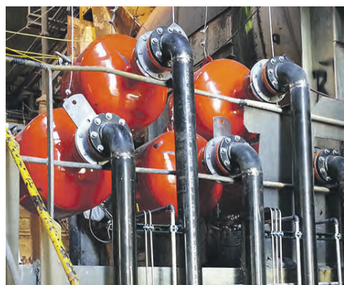
4.5 inch (11.5mm) pipes lead down to holes drilled into the concrete floor, then continue under the subfloor.
