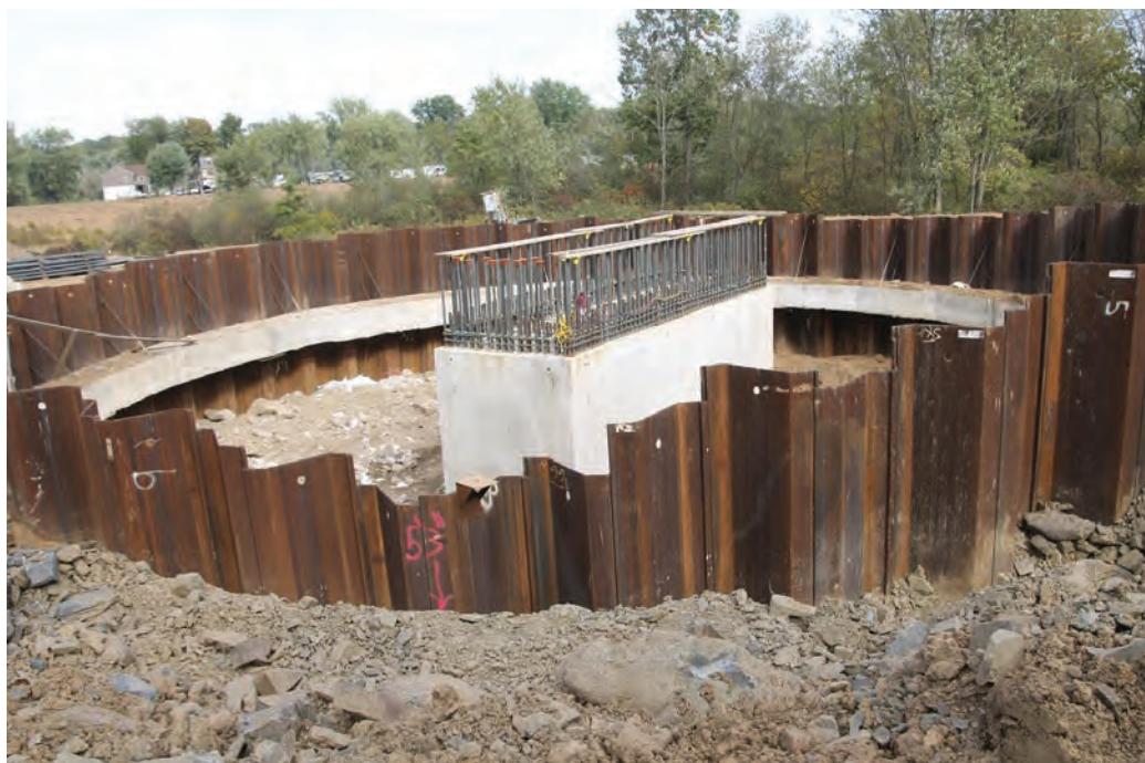
Rising from an excavation 20 feet deep, the concrete has been poured into a form over the rebar structure that will strengthen the first 28-foot section of this bridge pier. Soil has been filled in around this base.
