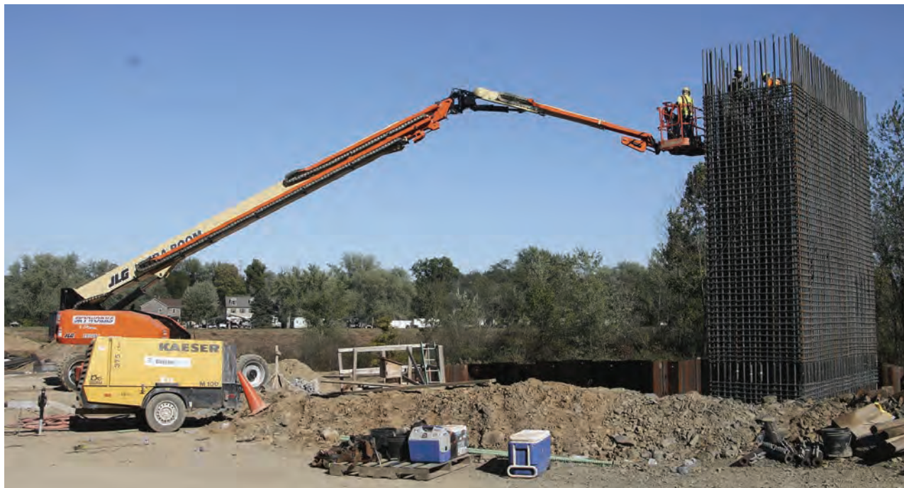
This intricate rebar structure will go to the base of the bridge pier, 20 feet below ground level. A JLG™ Ultraboom manlift demonstrates its secure reach and flexibility as it delivers another worker to a site near the top of the structure.
