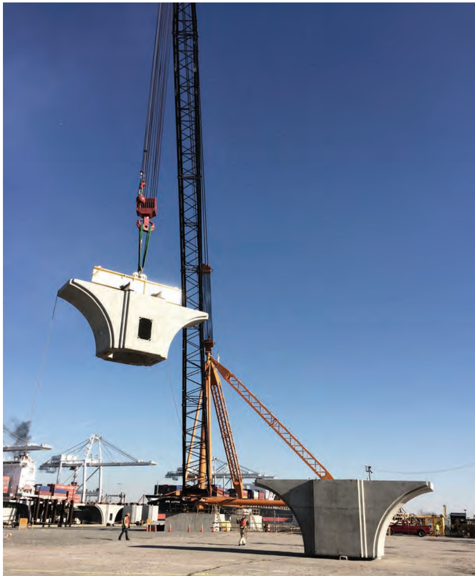
An American Cranes S-60 lifts pre-cast concrete bridge segments at the Bayonne Bridge project in New York.
