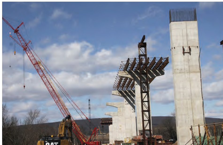
By mid-March 2018, several bridge piers had reached their full height and the first girders could be placed on Span 6.
