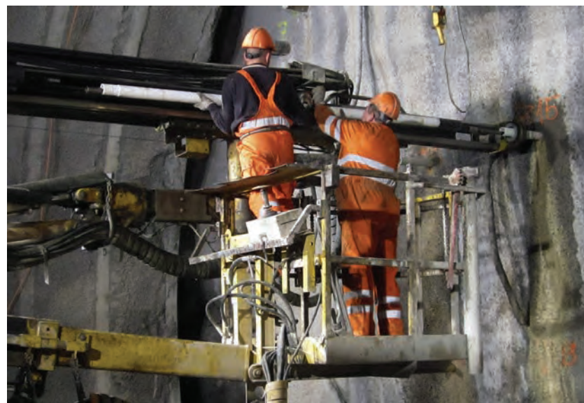
Robit's rods are manufactured using carefully selected hollow drill steels, with the drill rods ensuring maximum strength with long thread life.
