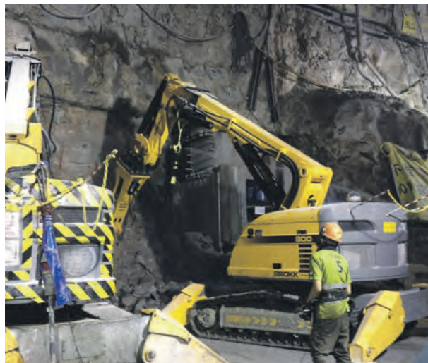
A Brokk robot working with an Atlas Copco breaker on a tunnel face.
