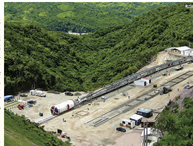
A project in San Juan de la Maguana used Herrenknecht equipment for a tunnel project of almost 15 feet in diameter (4500mm).
