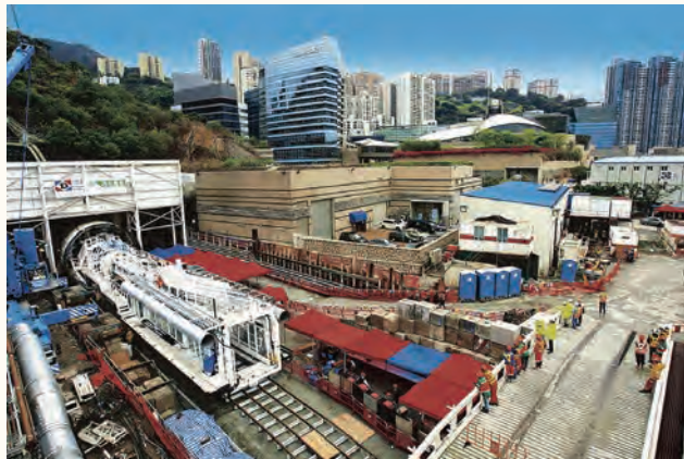
A Herrenknecht Double Shield TBM was used for an urban sewage tunnel in Hong Kong with a diameter of over 27-feet.
