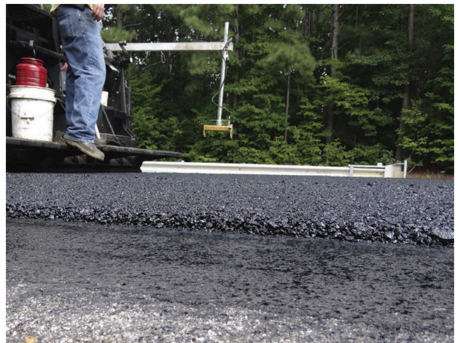
The laydown included the milling of existing pavement at a height of 2.5 inches followed by the placement of a surface mix and the OFGC.
