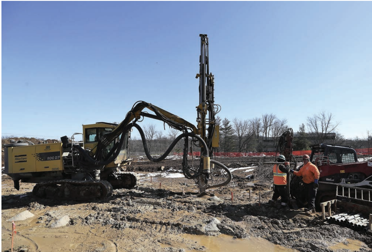
Drilling subcontractor Brubacher Excavating used an Atlas Copco ROC D7 Drilling Rig to pre-drill 3.5-inch-diameter holes and install temporary steel casing.
