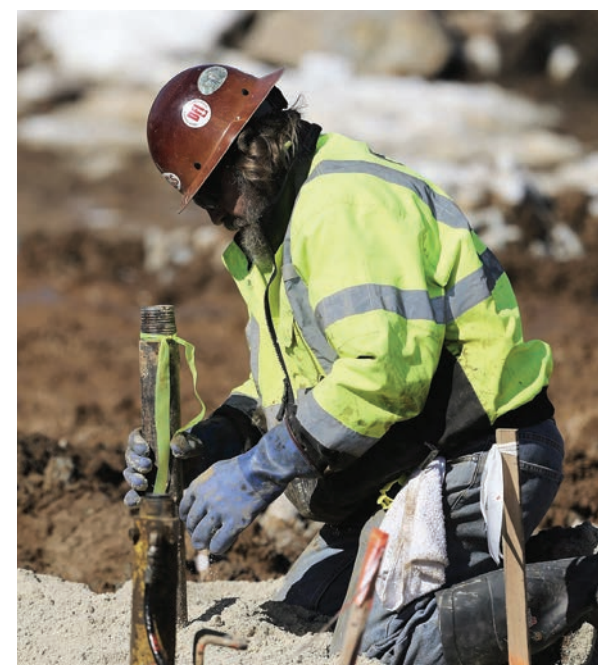
Mike Miluski checks the temporary casing to prepare for grout injection.
