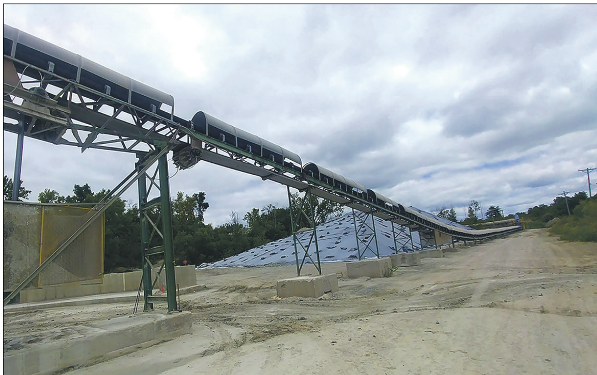
The 107-1 conveyor rises 20 feet (6 m) at its mid-section.
