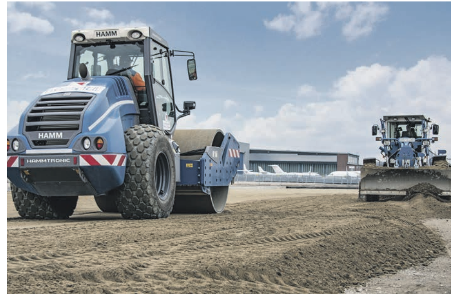
The hydraulically bound base at Cologne/Bonn Airport was compacted by a Hamm H 16i compactor.
