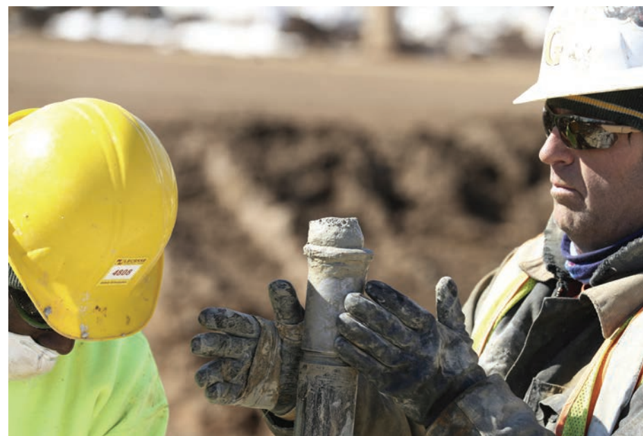
Backpressure from the soil forced the grout out of the pipe.
