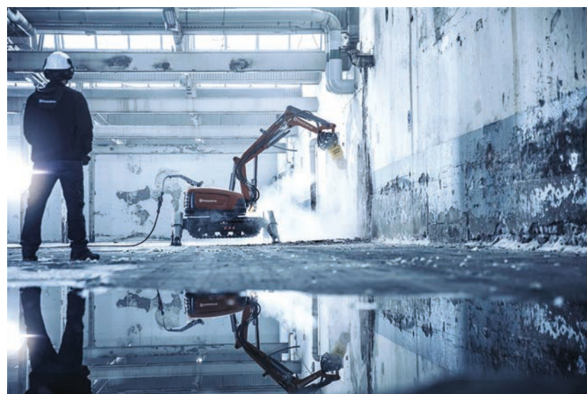
The robot uses a water based-dust control system which is ideal for dealing with airborne contaminants.
