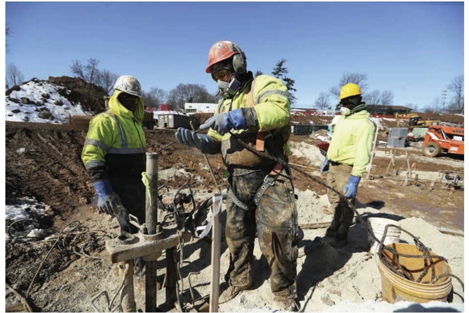
The 2-inch inside diameter temporary casing was equipped with a bullet point on the bottom that was intentionally knocked out by yanking a rope from ground level to avoid clogging the pipe with grout.
