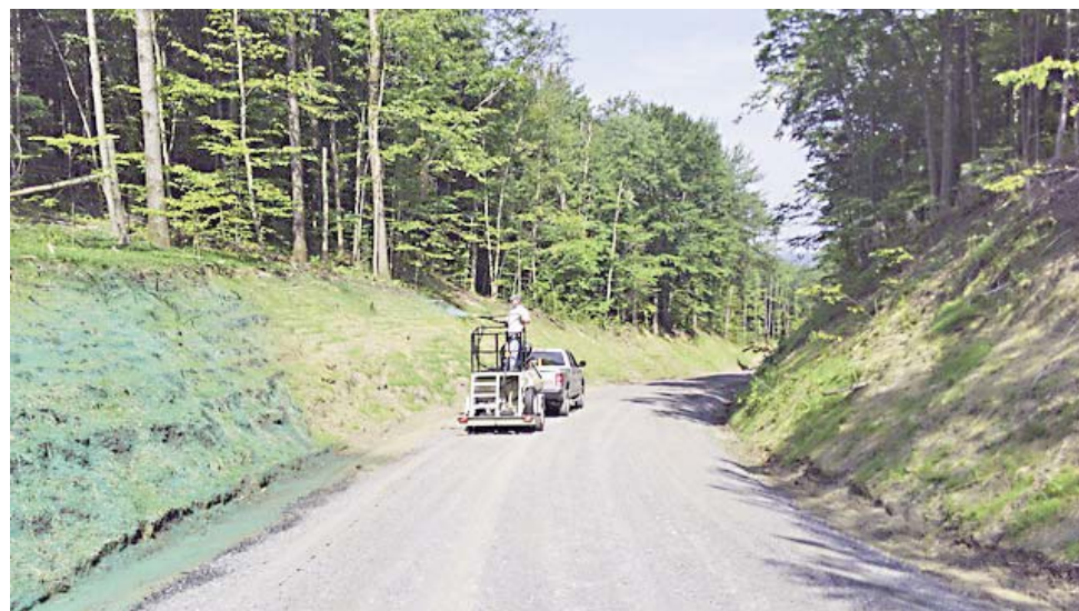
Hydroseeding along Burt Road, in the Town of Norway, was done last year by the Herkimer County SWCD. For more information and hydroseeder availability for 2018 stop in or call the office at 315.866.2520 Ext 5.
