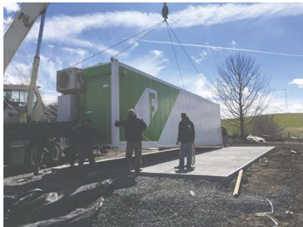
Freight Farm Leafy Green Machine being set in place
