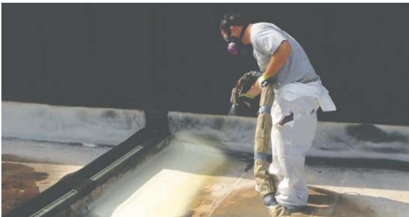
Applying spray foam on top of the roof structure creates a seamless waterproof layer that provides more complete, failsafe waterproofing than other roofing options.
