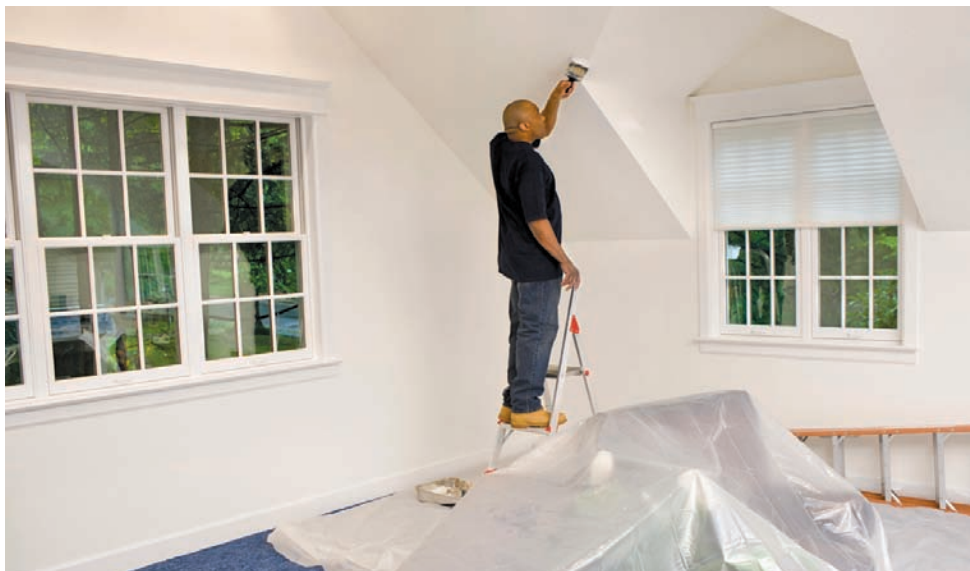
It pays for homeowners to address stains on their ceilings as soon as possible.
