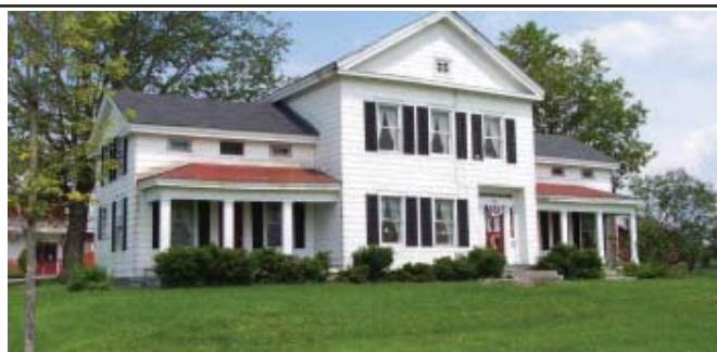
(112) SPRAKERS: CUSTOM KITCHEN. REBUILT CHIMNEY. 1500 GAL SEPTIC. NEW WELL AND PRESSURE PUMP. HEATED OUTBUILDINGS. ENDLESS POSSIBILITIES FOR ANY TYPE OF BUSINESS. MOTIVATED!
