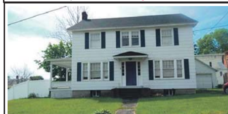
405: 7 Spring Street, FORT PLAIN: This Colonial home has hardwood floors throughout. The heating system (hot water) and roof are about a year old. Upstairs there is a new deck off the large master bedroom with a nice view. The second bedroom was once two bedrooms and could easily be converted back to two. There is a charming alcove at the top of the staircase. A large porch covers the entire side of the home. The yard is fenced in. There is a two-car detached garage. Asking $70,900
