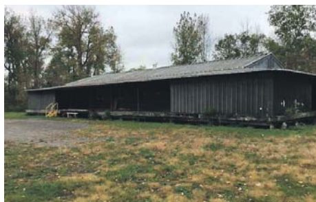
217: 0 Otsquago Club Road, FORT PLAIN : Perfect for anyone who needs land and or a building for storage. The warehouse alone is 2,160 square feet. Platform dock 1,896 square feet. One cement block building for electric/heat and the 3rd metal shed for tools, storage, etc. Recently was used by a propane company and also used by a snow mobile club. Asking $49,999
