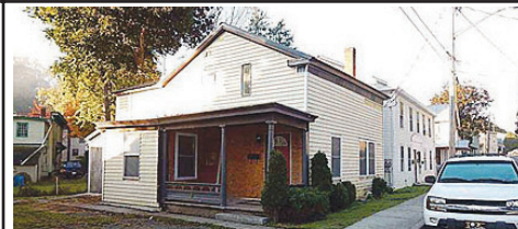
533: FORT PLAIN: From the roof to the furnace, everything is updated. New kitchen w/white cabinets and updated appliances. Lg living room with recessed lighting. Formal dining room with new flooring. Partial bath downstairs w/tile flooring and W/D hook-up. Remodeled full bath upstairs. Home is well-insulated w/reasonable heating costs. . . . . Asking $49,000
