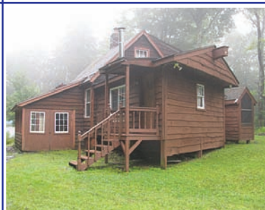
GLOVERSVILLE MLS 201417938 $79,900 LOOKING FOR A GET-A-WAY SPOT but don't want to break the bank? This camp is in great condition and very close to the lake.
