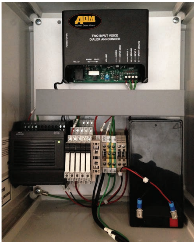
Asphalt Drum Mixers Inc.'s call box notifies operators of an event at the plant. The call box can be tied to most plant systems, but it is most often used to monitor asphalt tank temperature.
