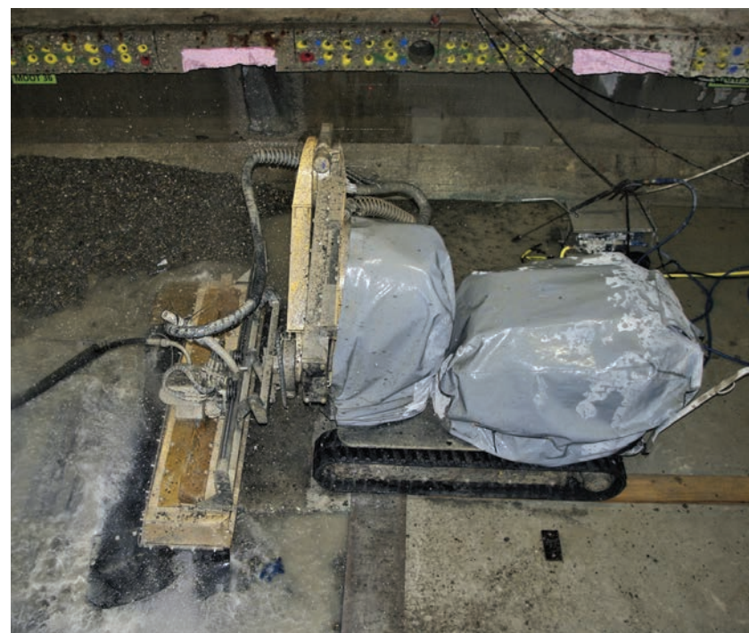
A hydrodemolition robot from Conjet at work on a bridge project in the Netherlands.
