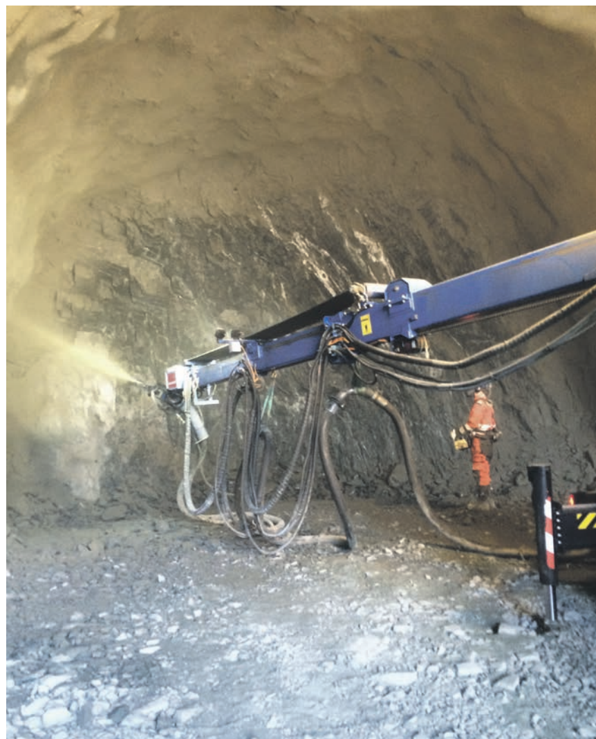
Shotcreting the tunnel lining with product derived from rock tunnel.
