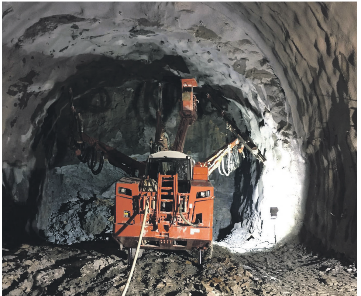
A Sandvik tunneling jumbo at work on the Contract 6 road tunnel.
