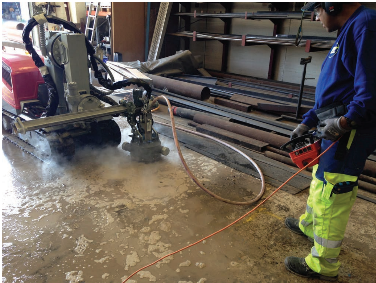
The Aquajet Systems AB Rotolance effectively cleans, removes and roughens concrete surfaces, leaving a better bonding surface for new concrete or alternative materials.
