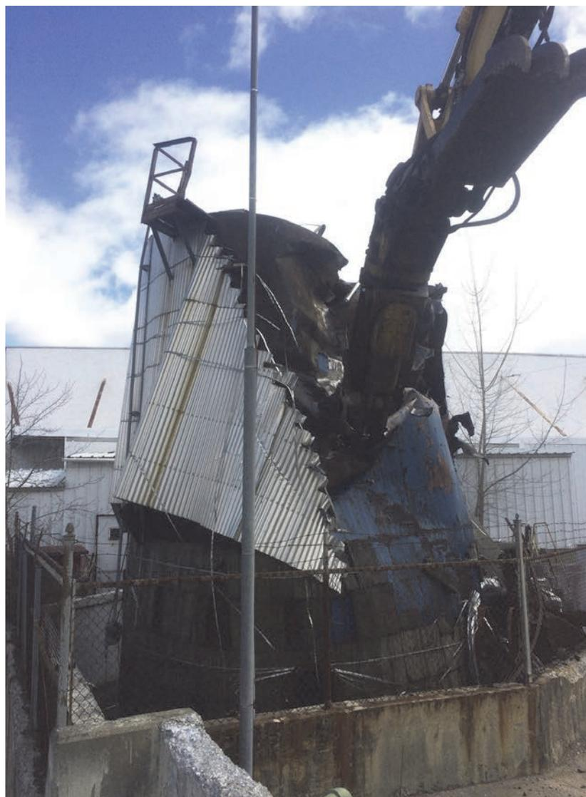
Ralph Hotaling, lead equipment operator, nears completion of taking down the 50,000-gallon steel tank.
