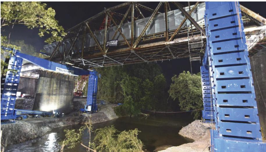
The team transported the new railroad span onto the old bridge using 24 lines of Goldhofer E-Steer SPMT with 90-degree traverse movement capability to align the span with the railroad track.
