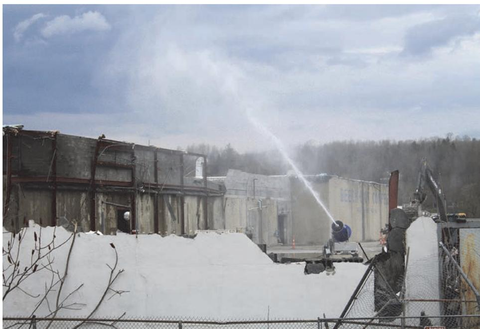
Dust control is continuous during demolition.
