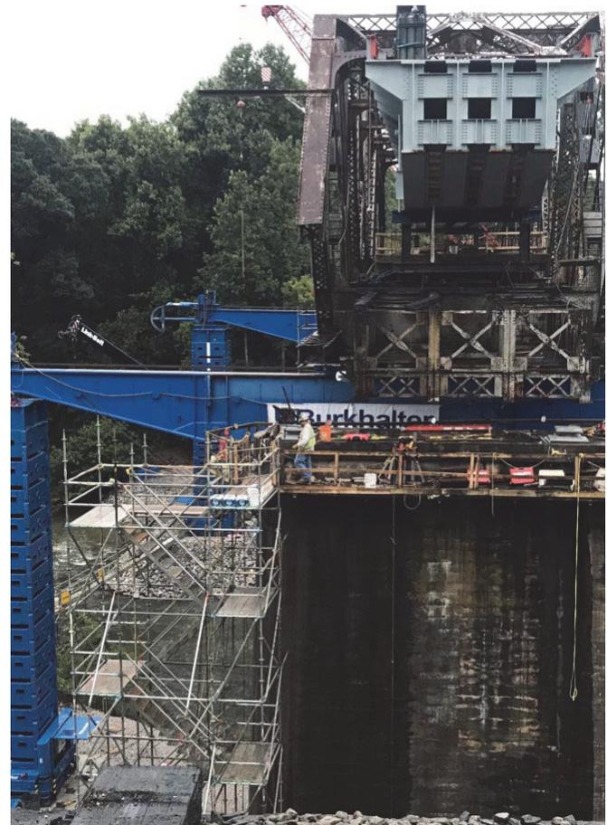
Upon alignment, the new span was then lowered into place with Enerpac's BPU-750 jacking system while simultaneously lowering the old bridge.
