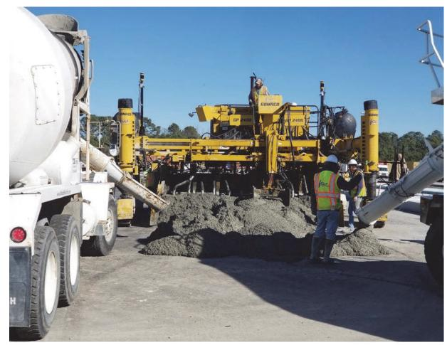
The system has machine-control positioning zone-laser receivers with integrated GPS antenna mounted on the rear of the paver. Other components on the paver include the machine control GNSS receiver and slope sensors to control the front or "draft" of the paver.
