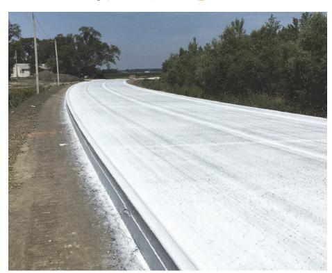
The Topcon Millimeter GPS paver system appears to help with paving accuracy — both in material usage and concrete lay down.
