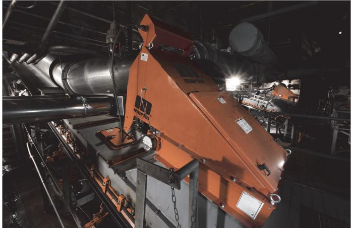
An integrated air cleaner is a small, independently-operating unit placed at the dust generation point.
