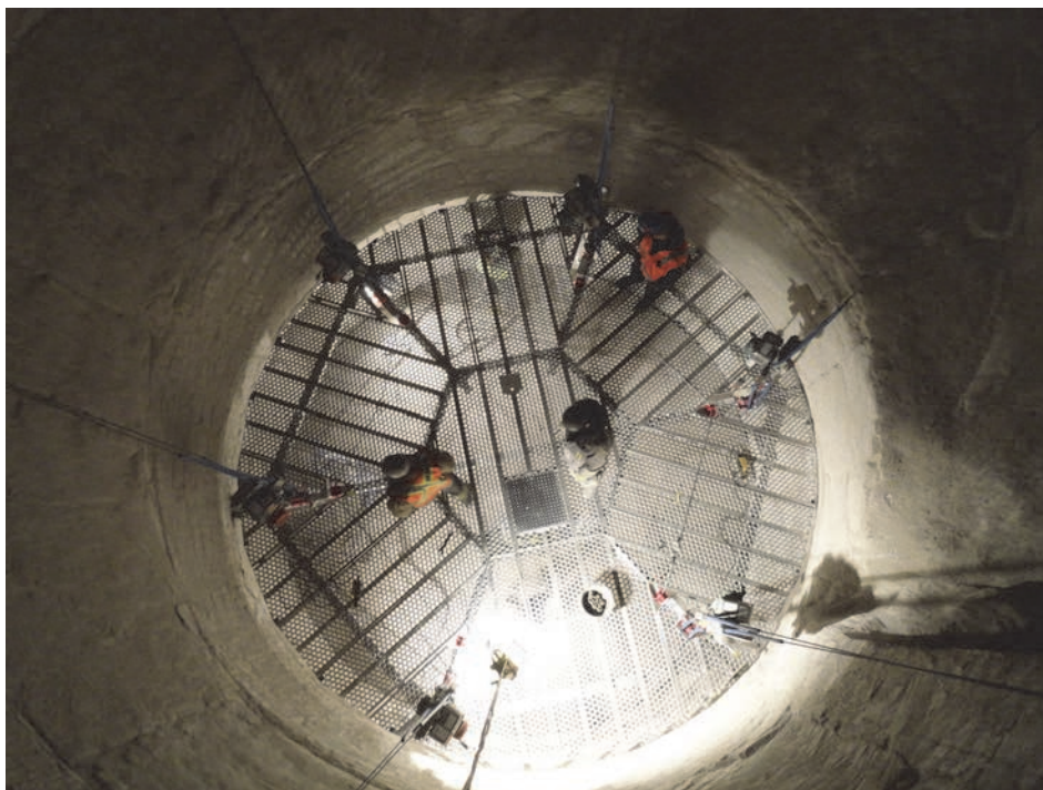
The 22-ft diameter EZ Lift Suspended Platform, constructed of high-strength 6061-T6 aluminum, offers a net load capacity of 6,000 lbs (2,722 kg).
