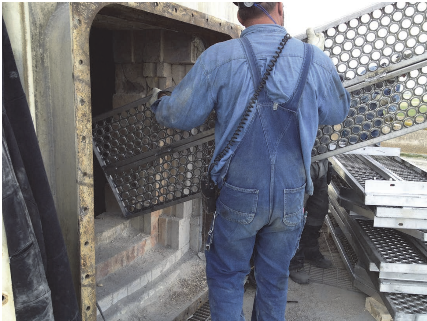
Left: Each section of the EZ Lift suspended platform weighs less than 45 lbs and effortlessly fits through the kiln's 54"-high by 36"-wide door.
