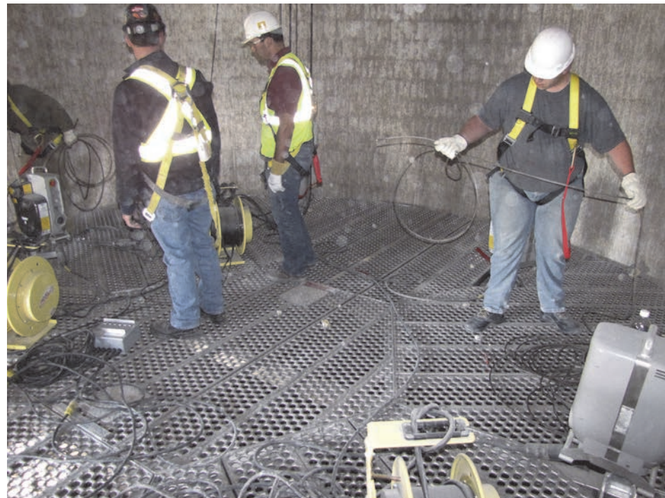
Above: The 360° accessibility provided by the EZ Lift means crews can quickly complete more thorough inspections, decreasing downtime.
