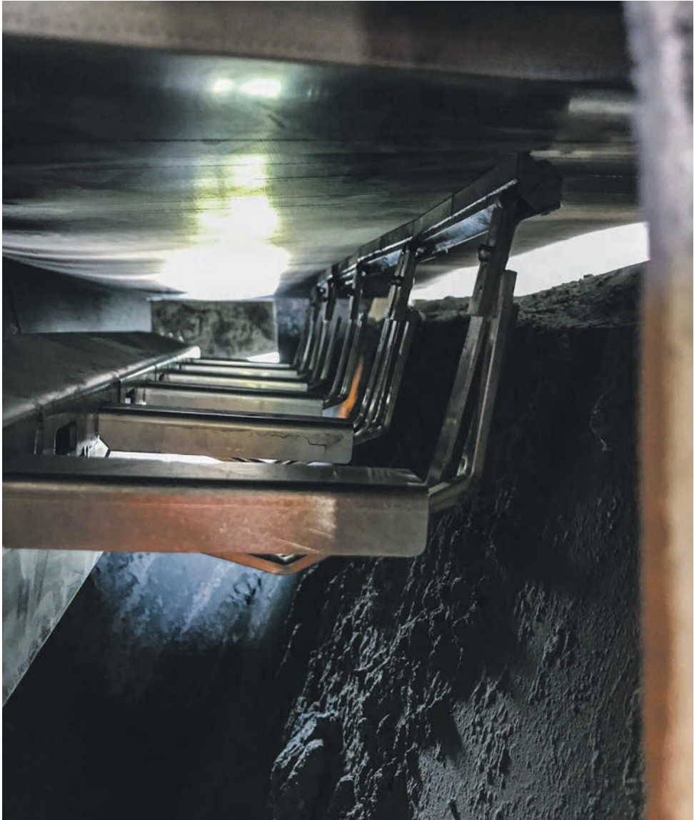
The new secodary belt cleaner is engineered to minimize maintenance and conveyor stoppages.
