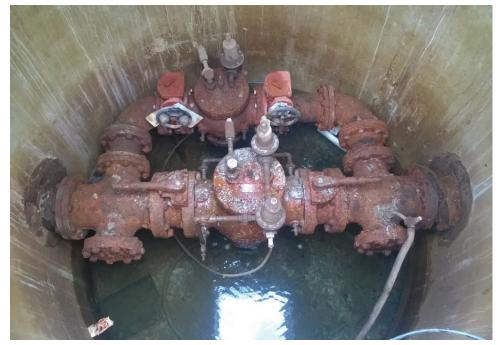
Near zero-gap flange spreading is further complicated by tough conditions and space restrictions in this pit.
