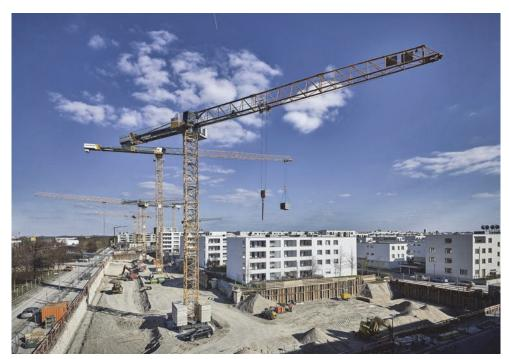
Many parts on the upper elements of the crane are optimized for transport and assembly with the new EC-B compact head, boom and trolley being lighter than their predecessors.
