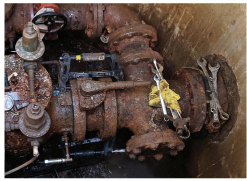
Two Equalizer SG4TM Mechanical Flange Spreaders facilitate replacement of two isolation valves safely and efficiently.
