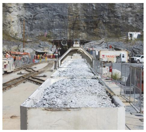
The relatively small diameter of the tunnel in the project, coupled with the grade and the use of muck haulage, made sizing and balancing all aspects of the equipment a particular challenge.
