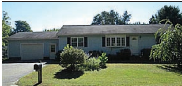
204: ST. JOHNSVILLE: Modular home w/nice fenced yard and great neighborhood. Attached garage. Formal dining room. Wood floors, except kitchen. Full basement and attached garage. Easy home to heat. Vinyl sided exterior. . . . . Asking $119,900
