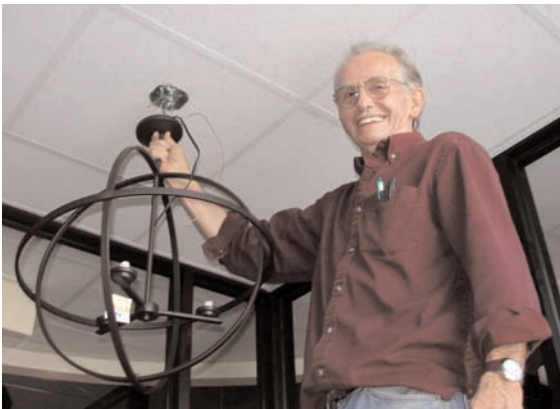
Ruby & Quiri's Master Electrician Jack Davin installs a lighting fixture as the finishing touch in the store's main entryway.
