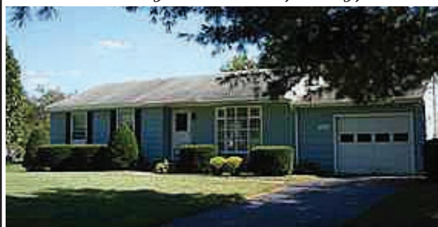
264 Co. Hwy. 154, Town of Mayfield
