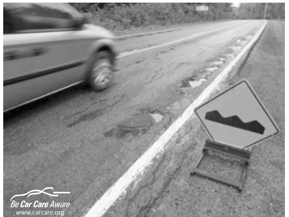
This year's brutal winter weather has resulted in an unprecedented number of potholes appearing on roads and highways across the country.
